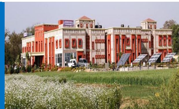
Administrative building cum Laboratory, ICAR- RCER, Patna
